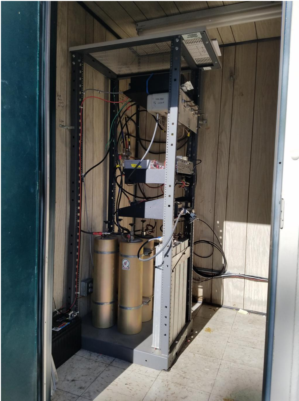
Looking in the door. DSW backup battery on the left; SMRA backup battery in far corner (not shown)
