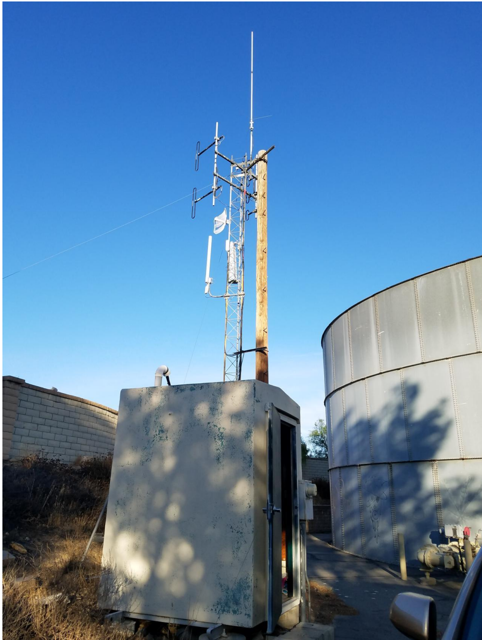
A view of the building, tower, antennas and water tank. The building is only used for ham radio now. On top of the building is the cableway.
