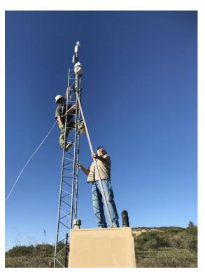
We found that while the tower is very secure, it's not secure enough to provide a stable video platform. So on MLK Day (Jan 21) we undertook with the property owner's blessing a project to add bracing to the tower. Photos show the work party, consisting of me, W6BI, Eric KE6MLF on the tower, and Dave KM6FQ (ground assistant and photographer).
